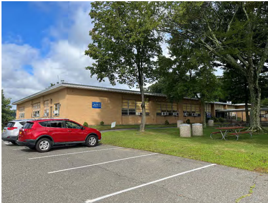
Don Bosco Retreat Center building, showing the southern and eastern facades.
