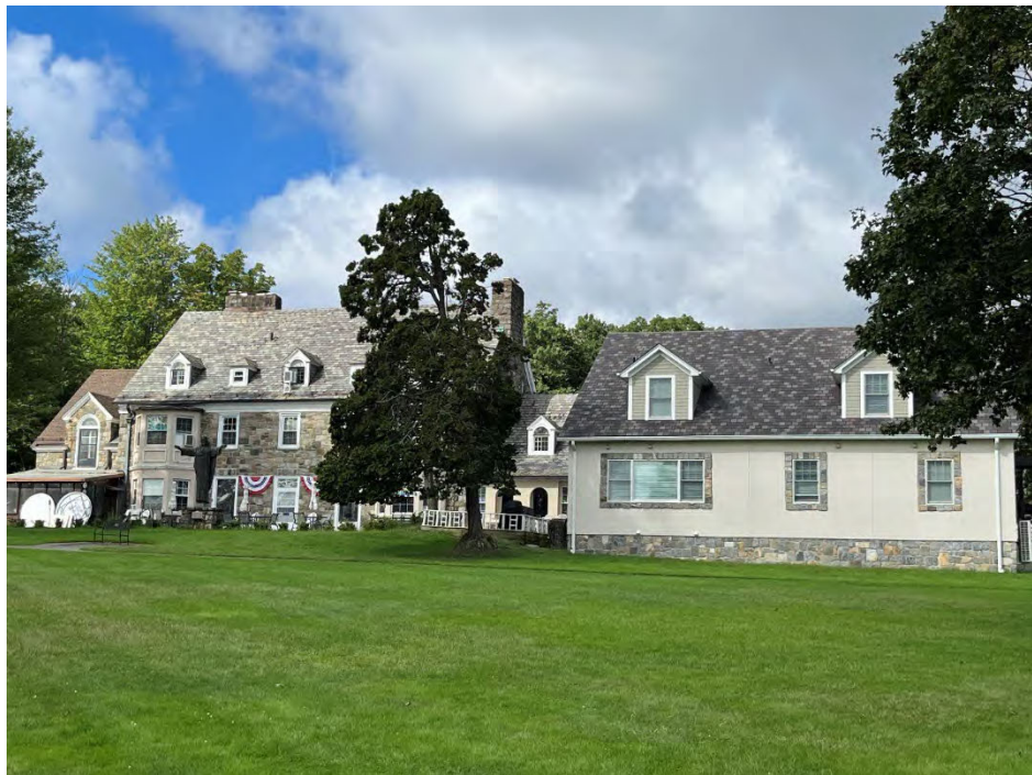
Residence building, photo taken showing the Eastern façade. It sits approximately 1300' North of the proposed project area and there is no line of sight.
