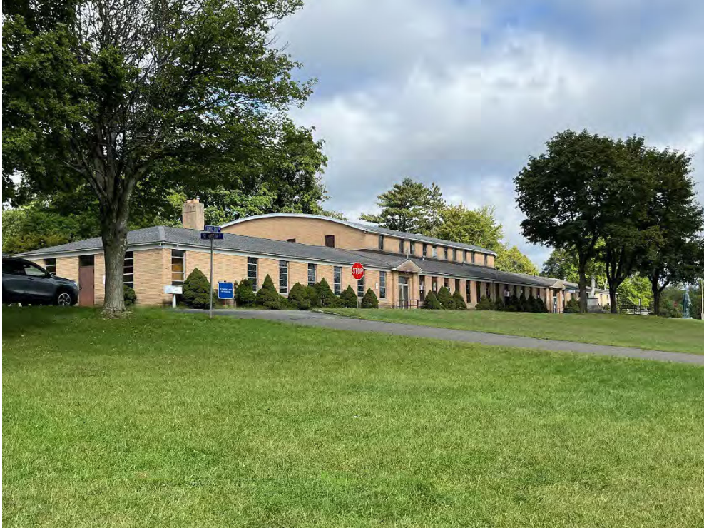
The St. Dominic Savio Youth Center, as seen from the Southeast. There is no line of sight to the project.
