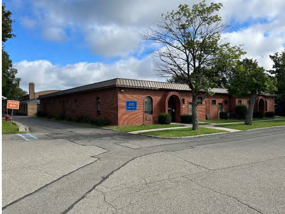
Main Office building, showing Southern façade. As one exits the doors, one would have a limited line of sight to the proposed arrays.
